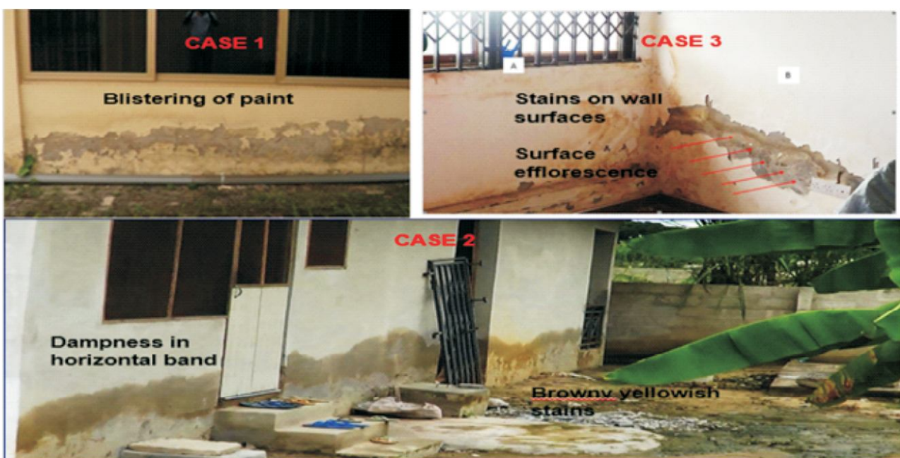
FIGURE 3.0: Symptoms associated with rising dampness
