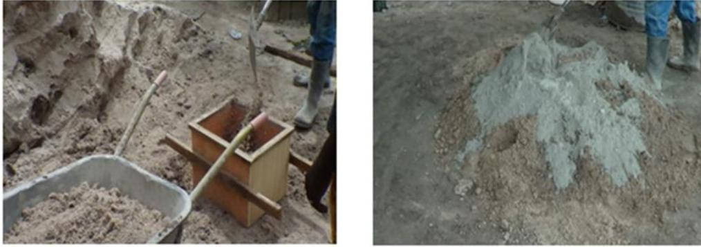
Figure 1. Volume batching of fine aggregates and cement
