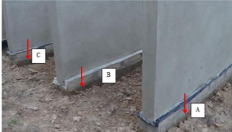
with three different DPCs - 0.15 mm thick (A), 0.12 mm thick (B) and 0.13 mm thick (C)
