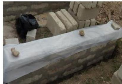
Figure 3. Diagrams showing how the polyethylene DPCs were laid
