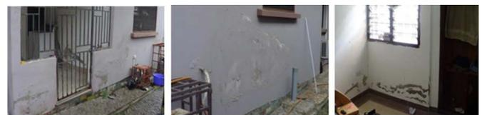
**Figure 3.** Some of the affected areas of the building identified during the visual inspection
