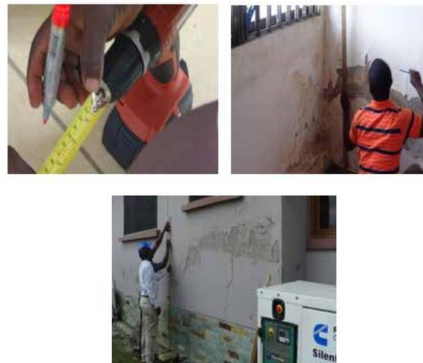
Figure 8. Measuring and drawing the grids using the tape measure and light wooden batten
